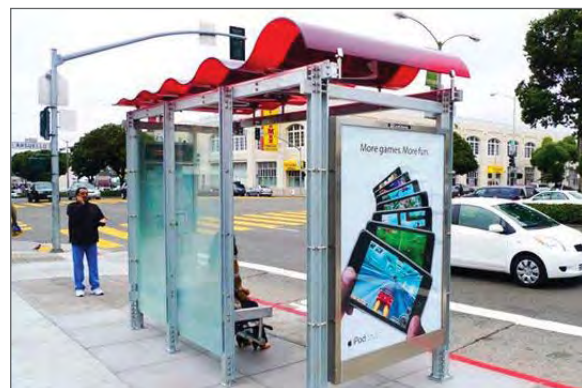
Solar Intercom, LED Lighting, and WiFi
